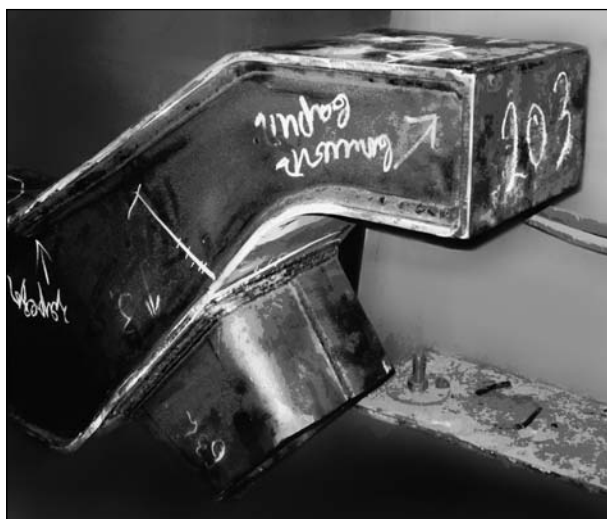
Fig. 3. Place of welding on lever bracket to bottom sheet
