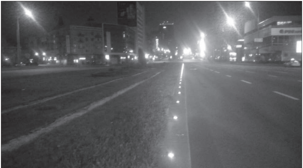
Fig. 2. Use of retroreflective elements developed at IIR of the NAS of Ukraine at the Victory Square in Kyiv
