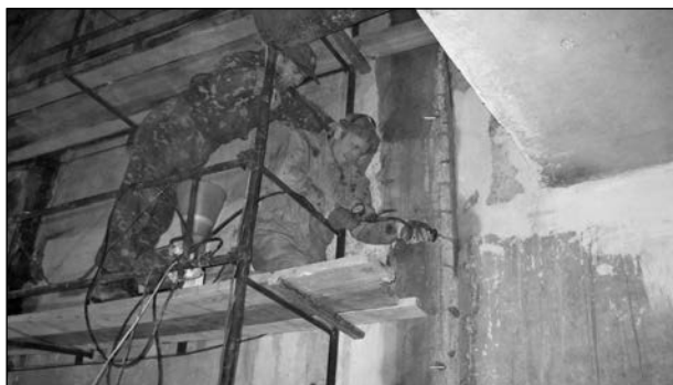
Fig. 9. Injection of polyurethane composites on Tashlyk HEPS
