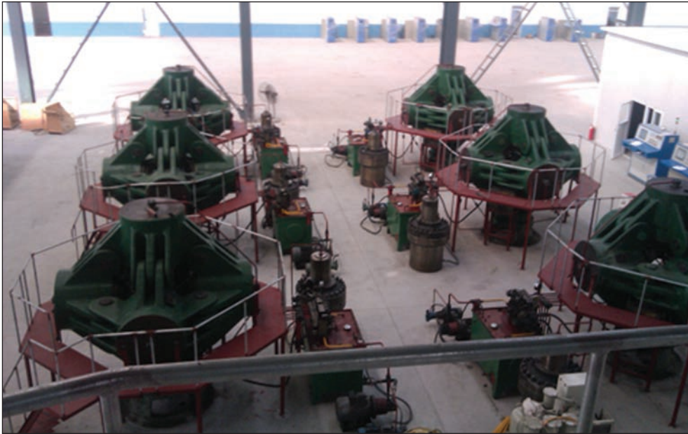
Fig. 6. General view of shop for the production of diamonds (equipped with 6-punch press CS-VII with a plunger diameter of 560 mm and load of 25 MN)
