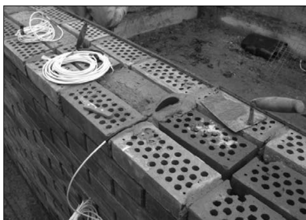
Fig. 6. Examples of sensors mounted in the walling of pilot passive-type house
