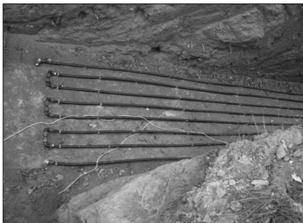
Fig. 13. Ground–water 8-wire heat exchanger
