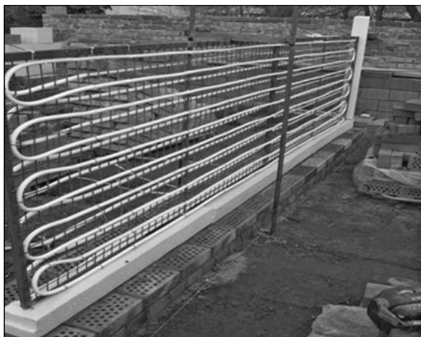
Fig. 19. Heat exchanger imbedded into the concrete partition wall
