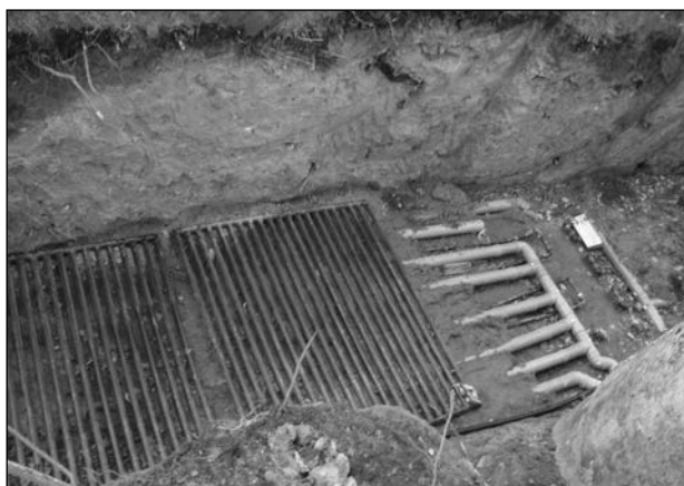
Fig. 15. Three-section multi-pass ground–water heat exchanger
