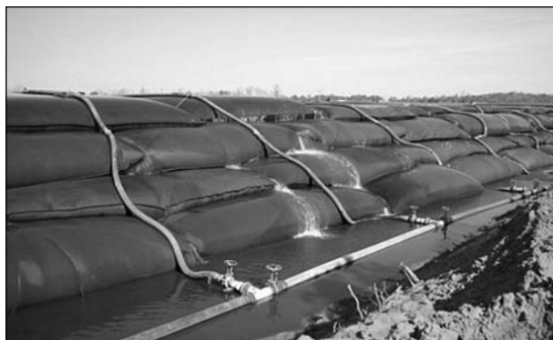
Fig. 1. Cascade-like placement of Geotube containers
